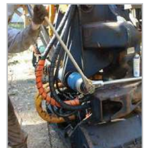
Torque multiplier used for machine nut tightening
